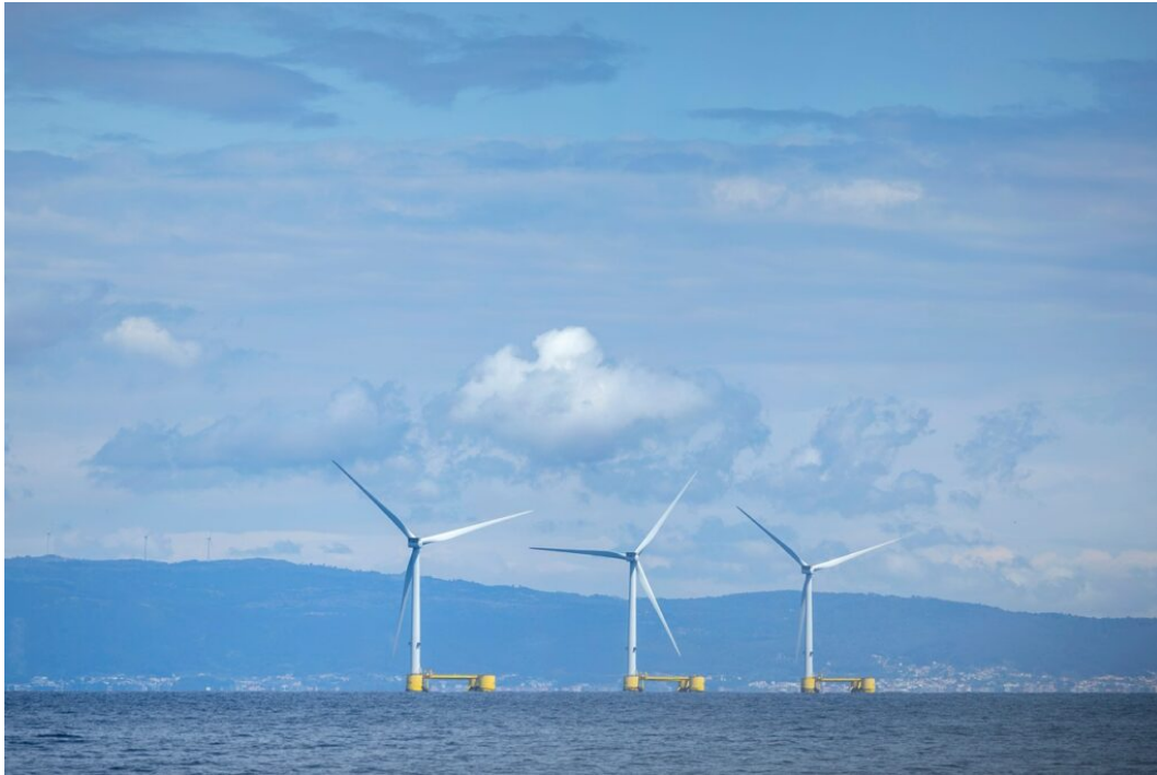
Figure 25: WindFloat Atlantic pilot project (Ocean Winds)
