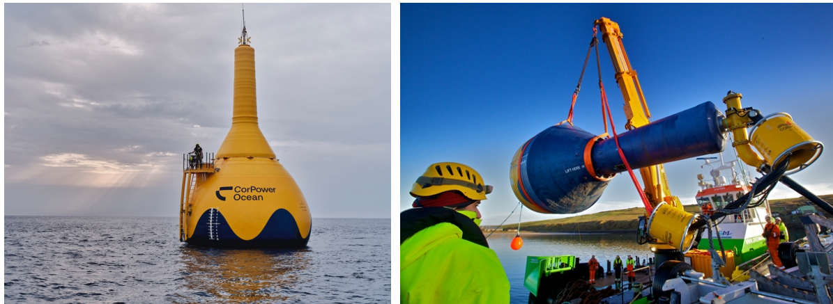
Figure 14: CorPower unit deployed at sea (Ocean Energy Europe, 2024) and in the process of deployment (The European Marine Energy Centre LTD, 2018)
